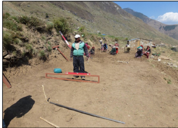
Photo 14: Use of camber template during training
