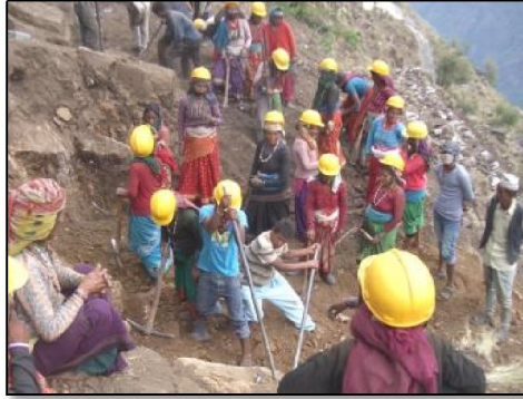
Photo 8: Rock-breaking team on CEP 2
