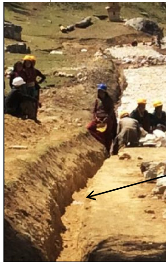
Photo 3: Side drain alignment
